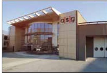
ASG INTERNATIONAL HEADQUARTERS - ITALY
