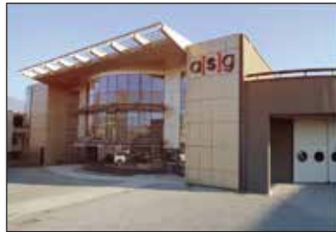
ASG INTERNATIONAL HEADQUARTERS - ITALY
